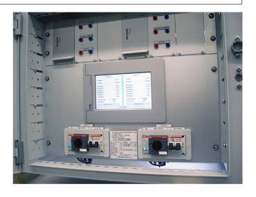
CORROCONTROL-2 can function as Output Regulator in existing and new impressed current cathodic protection systems.
