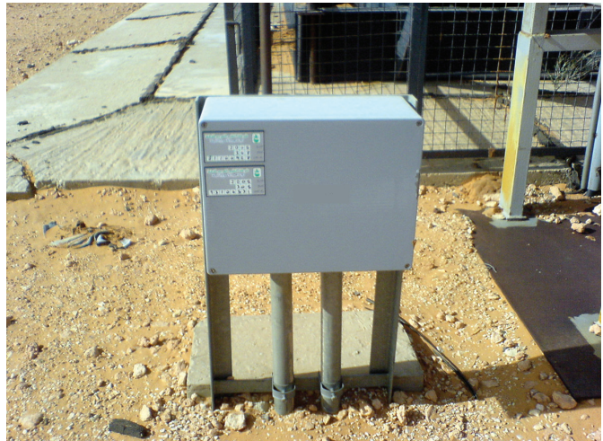
CJB with hot-dipped galvanised steel supports
