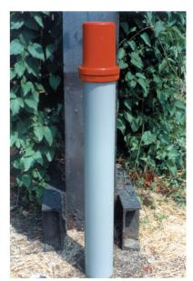
Anchor: polyethylene pipe on the lower post prevents removal.
