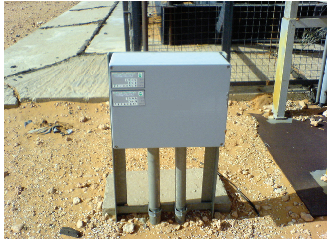
CJB with hot-dipped galvanised steel supports
