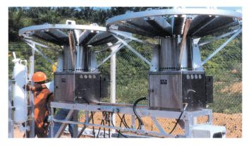
Natural gas pipelines are often protected with current supplied from thermoelectrical generators fuelled with natural gas tapped from the pipeline via suitable pressure reducing and valve arrangements.
